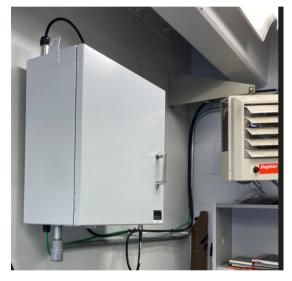
cable is secured along ceiling into control room where the M400 is mounted to the wall.
